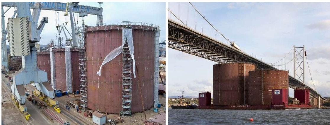
Figure 4 – Caissons during manufacture and shipping to the bridge site. (Photo: New Civil Engineer)
