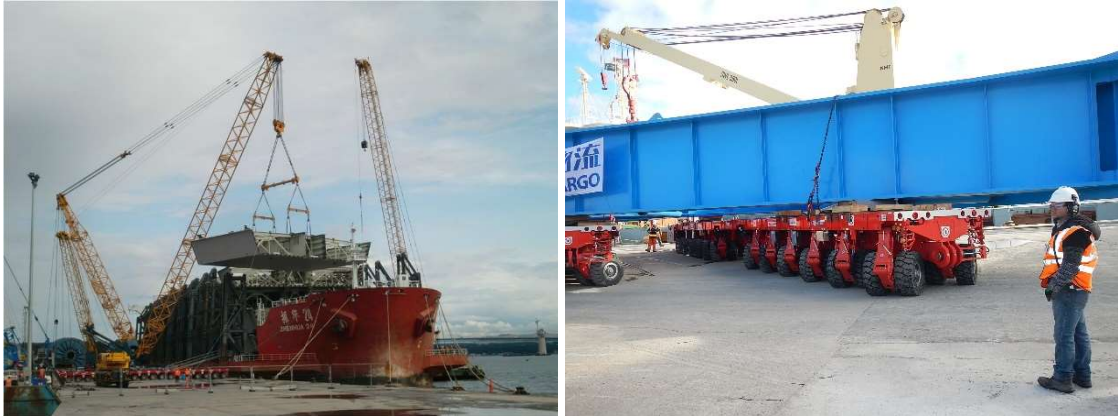
Figure 5 – Off-loading and yard transportation on SPMT's.
