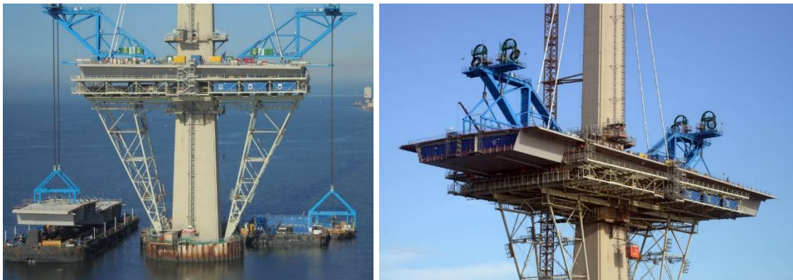
Figure 10 – First deck segment lifted by erection gantry, continuing with balanced cantilever construction.
