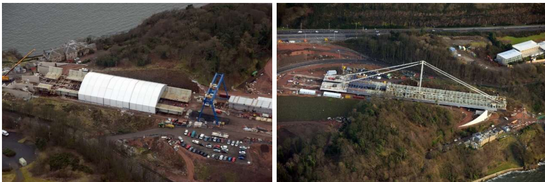
Figure 12 - North viaduct during assembly and launching.
