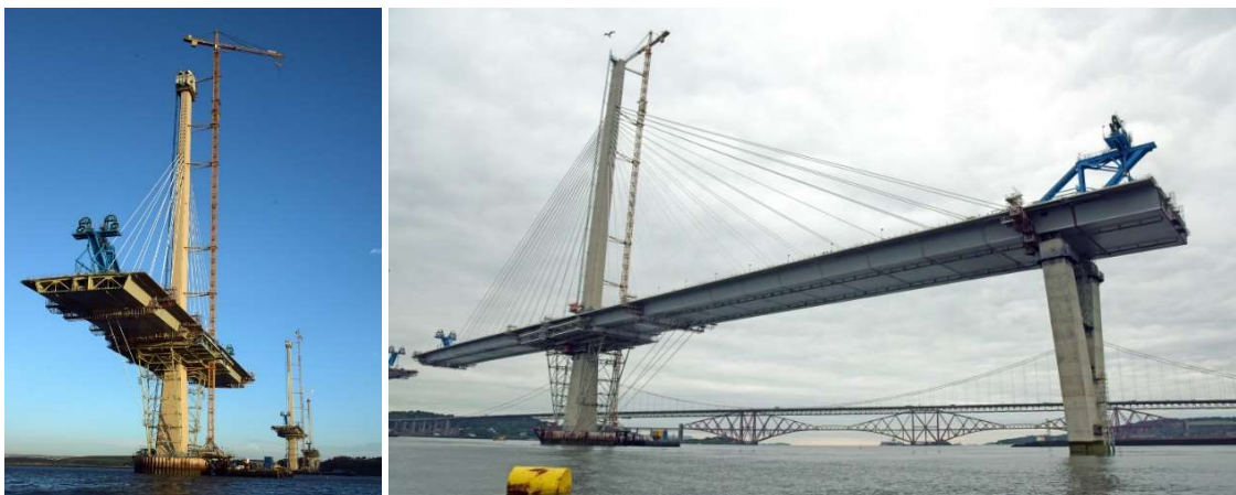
Figure 11 – Balanced cantilever erection from all towers up to the first pier pass.
