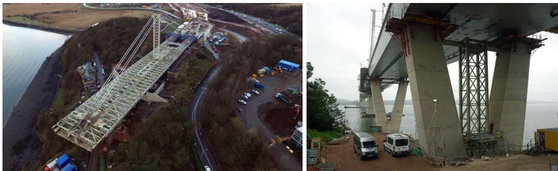
Figure 13 – North viaduct during assembly and launching.
